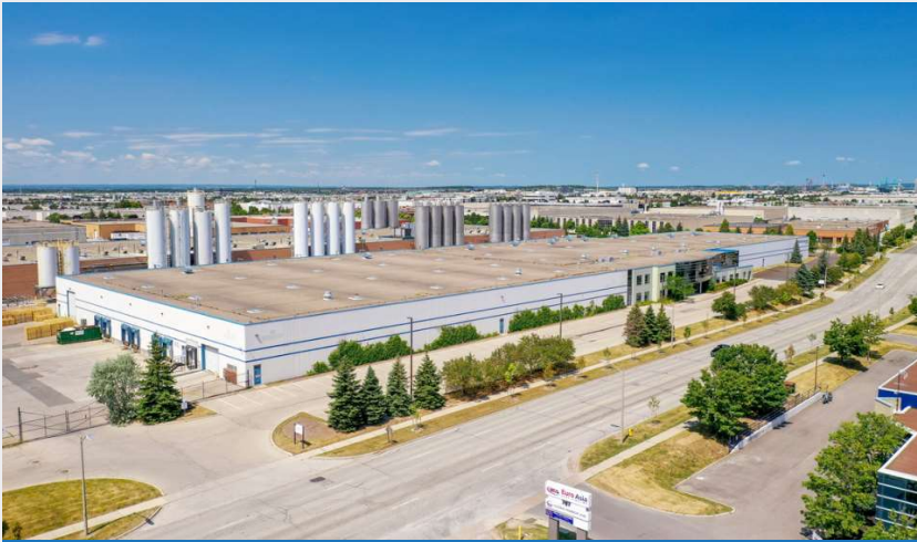
750 Creditstone & 121 Pippin Road, Vaughan
