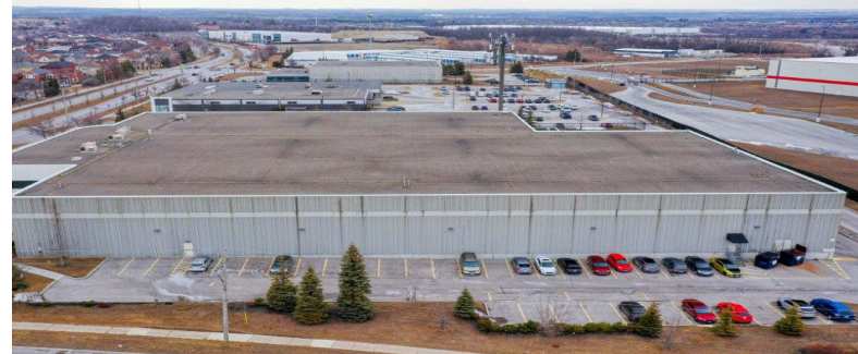
165 Harwood Avenue N., Ajax, ON
